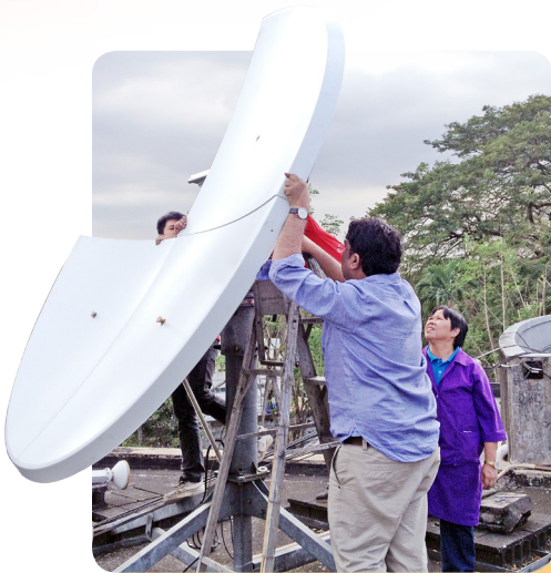
Installation of new VSAT antenna reflector at NDC-PH in PNRI for transmission of data to the CTBTO International Data Center
