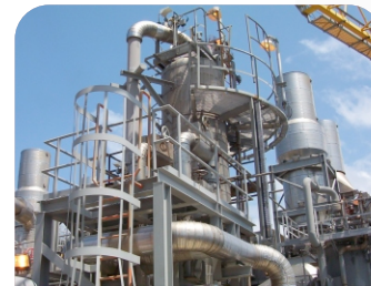
Gamma column scanning was used to diagnose process anomalies inside distillation columns at the Shell refinery in Palawan.
