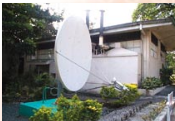
VSAT antenna that connects the N137 station to a satellite hub in Fucino, Italy to relay the data to CTBTO in Vienna.
